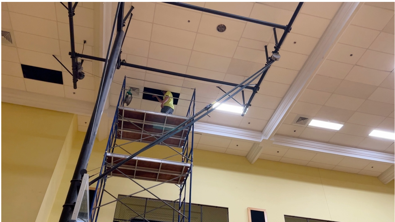
Providence School LED lighting installation.
