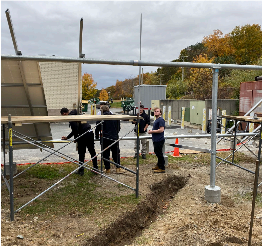
Students gain hands-on experience and install ground mount PV array system
