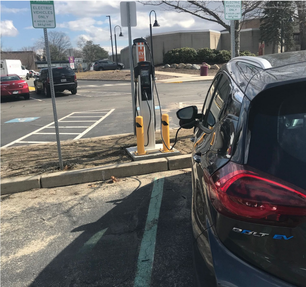
Installed five, dual port, level II electric vehicle charging stations
