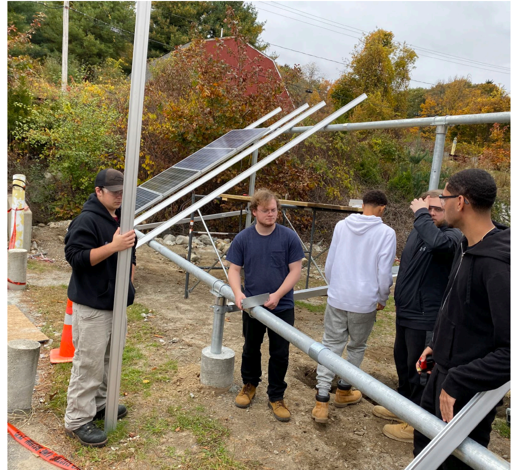
Students gain hands-on experience and install ground mount PV array system
