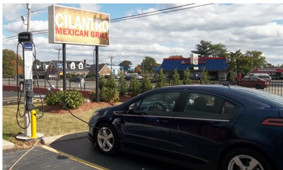
Public EVSE station, Cilantro Mexican Grill, Warwick RI
